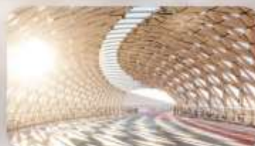
Atyrau Bridge Astana
