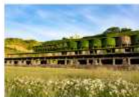
KITAZAWA FLOTATION PLANT
