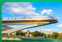
Floating Bridge Moscow
